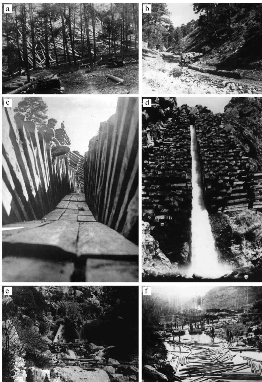
Fig. 8. Sequence of production and transport of black pine ( Pinus nigra ) railroad ties from forests in the Cazorla Mountains (south of Spain) down to the Guadalquivir valley. This manner of timber transportation was used until the mid-20th century. Source photos: Archivo Histórico del Museo del Ferrocarril de Madrid – Fundación de los Ferrocarriles Españoles.
