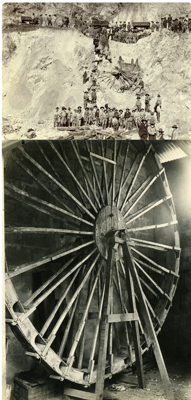
Fig. 4. Top: Roman waterwheel found in AD 1886 at the Rio Tinto mines in Huelva, south of Spain; the wood was dated by radiocarbon to 100–210 cal. AD; bottom: reconstruction of the waterwheel (source: Archivo Histórico Minero, Fundación Rio Tinto, pictures A-3-277 and A-3-279 respectively).
